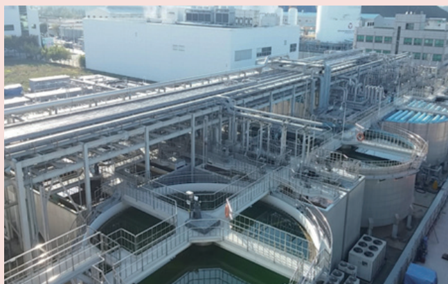
View of Wastewater Treatment Plant
